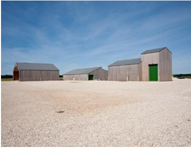
Building of the educational farm of the Sollier Agricultural College near Chartres (Eure-et-Loir) by Jean-Pierre Prin, Atelier Carré d'Arche
